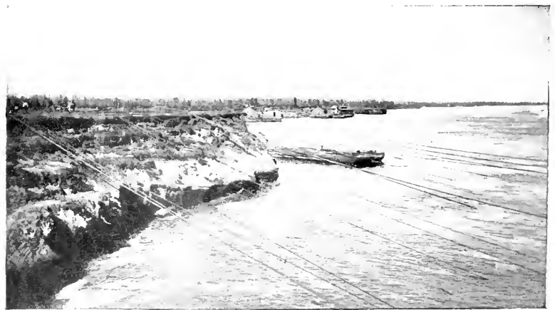
SYSTEM OF CABLES HOLDING MATTRESS DURING CONSTRUCTION.
